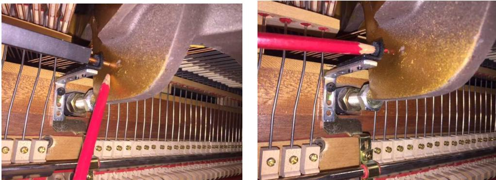
Figure 14 - Marking pivot rod horn hole location
